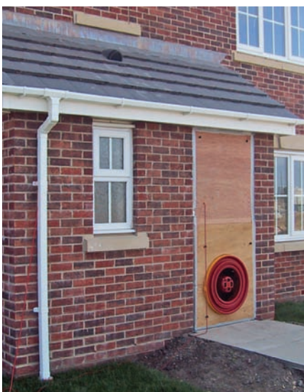
Blower Door Testing As part of the Code for its Sustainable Homes Assurance Scheme, Kingspan Century has developed air-tight details and systems and will undertake pre- and post-completion air pressurisation testing.
